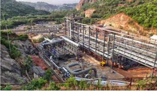
A view of ISPRL facility in Visakhapatnam
